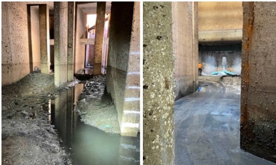
Up Close: Before and After Unit 3 Intake Structure
