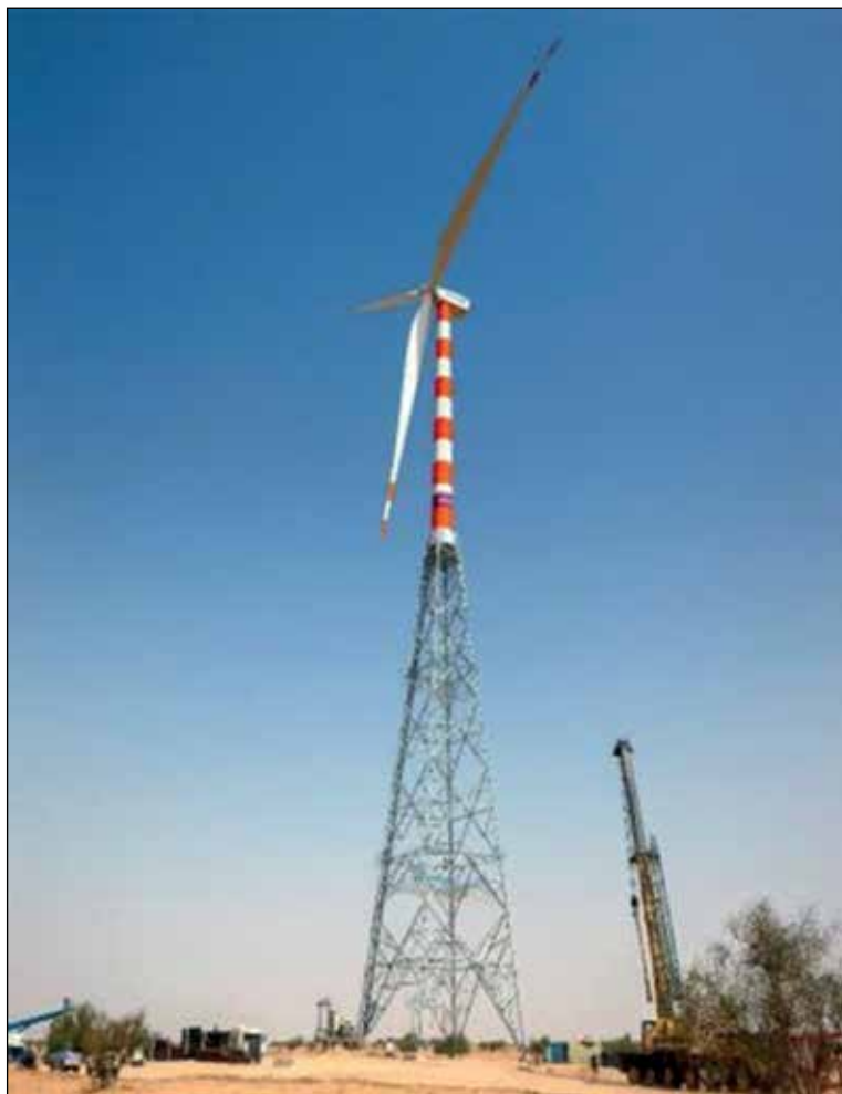
Fig. 10.23: Wind Turbine installed in Hybrid Tranche I-2X 195 MW Hybrid Project at Jaisalmer (Rajasthan)
