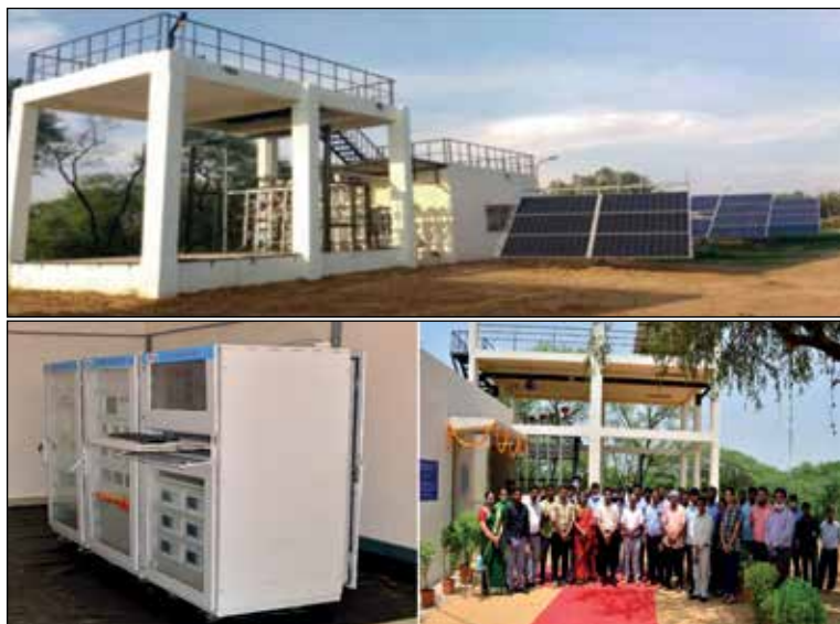
Fig. 10.4: Solar Water Pump Test facilities for up to 10HP (top), and for up to 50HP (bottom) at NISE
