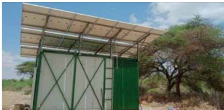
Fig. 10.6: A 5 MT solar powered cold storage with thermal energy backup application in Kenya
