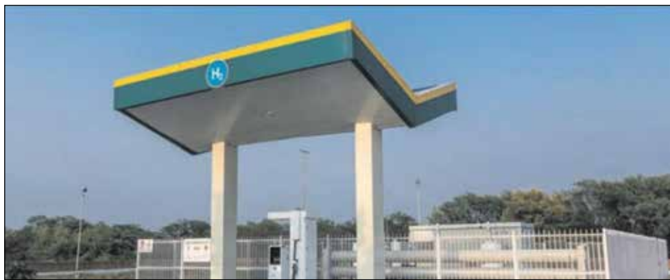
Fig.10.9: Hydrogen production-cum-dispensing facility at NISE
