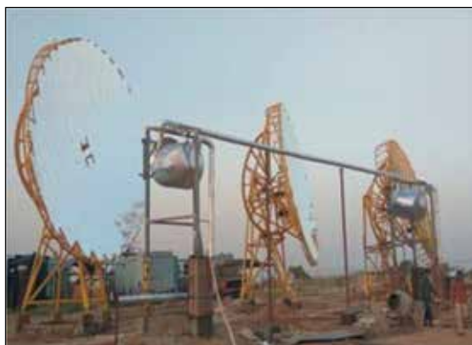
Fig. 7.18 Installation of cast Iron receiver with piping and Insulation
