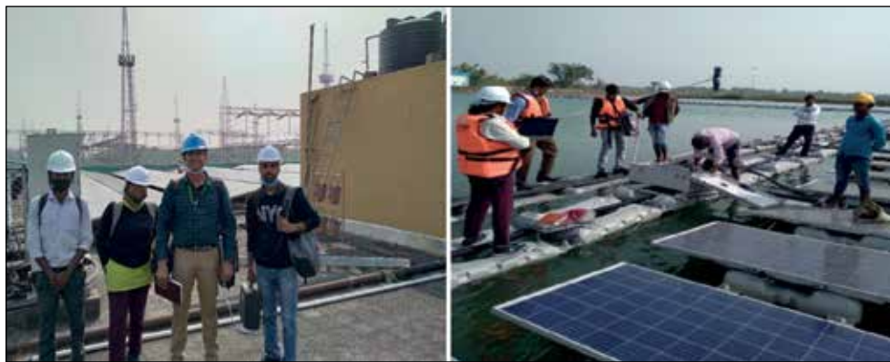
Fig. 10.10: Inspection and testing of PV modules in Rooftop (left) and Floating PV power plants
