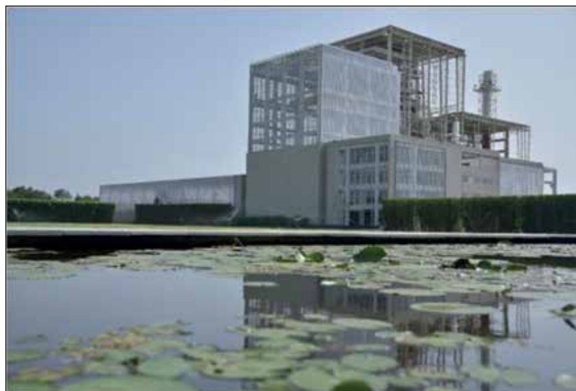
Fig. 4.6: 7.5 MW Power Plant based on Municipal Solid Waste in Jamnagar, Gujarat
