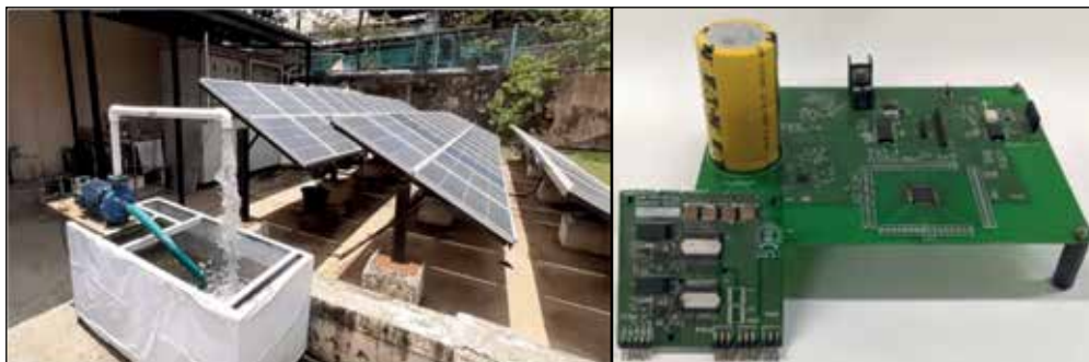
(a) Field testing of the developed BLDC pump (b) GaN based motor driver
