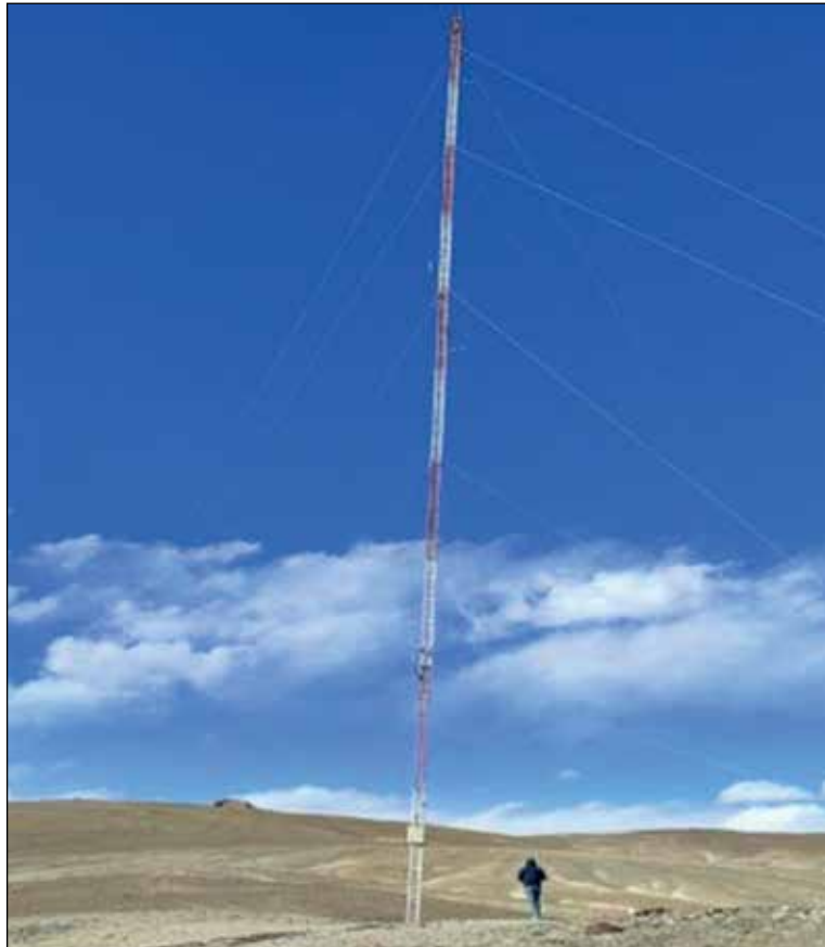
Fig. 10.12: 50 m wind monitoring station installed at Kargil
