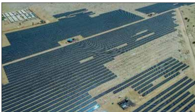
Fig. 10.24: 2x195 MW Project under Hybrid Tranche I at Jaisalmer (Rajasthan)
