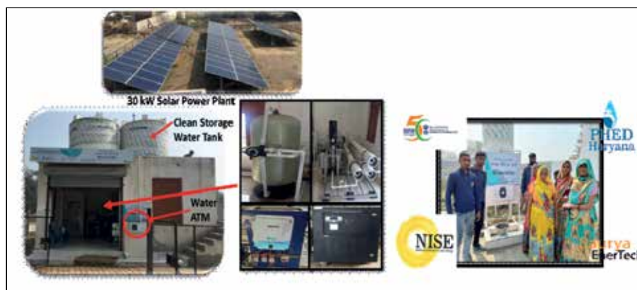
Fig. 10.11: IoT based Solar Powered Clean Drinking Water supply through automated dispensing installed at Faridpur village, Haryana.
