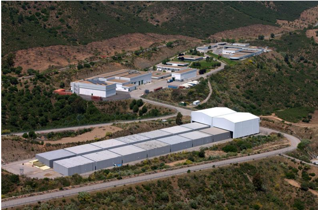
Figure 4. El Cabril Radioactive Waste Facility: The storage vaults are in the foreground, adjacent to two movable white roofs to cover each vault while being filled and sealed.
