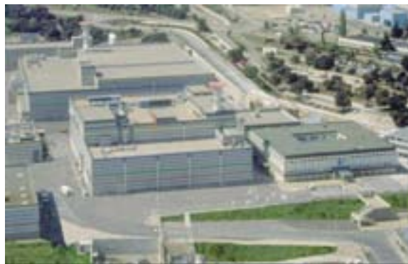
View of the MELOX plant.
