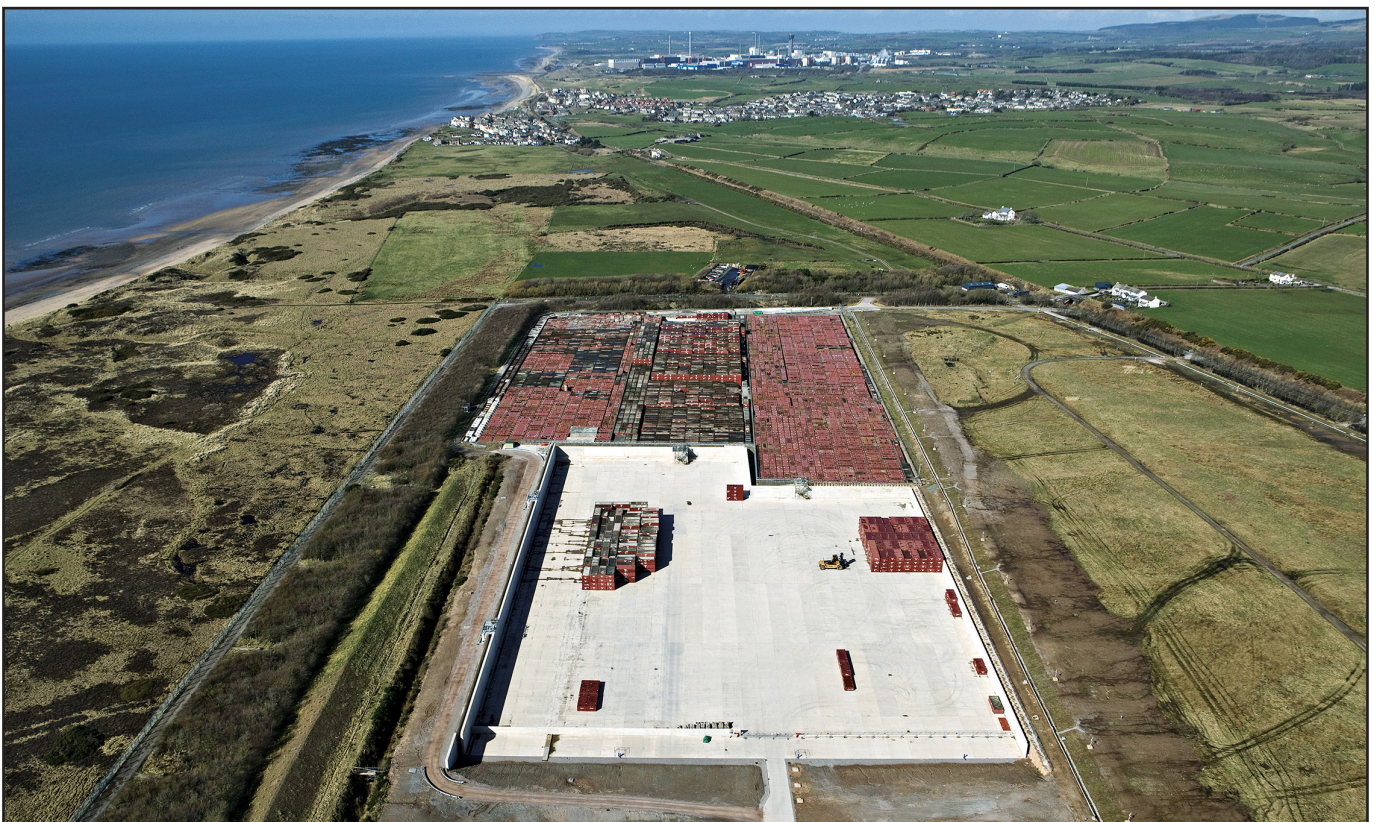
The Low Level Waste Repository in Cumbria, with Sellafield in the distance.
