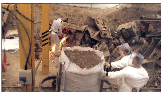
Clearing land contamination at Harwell
