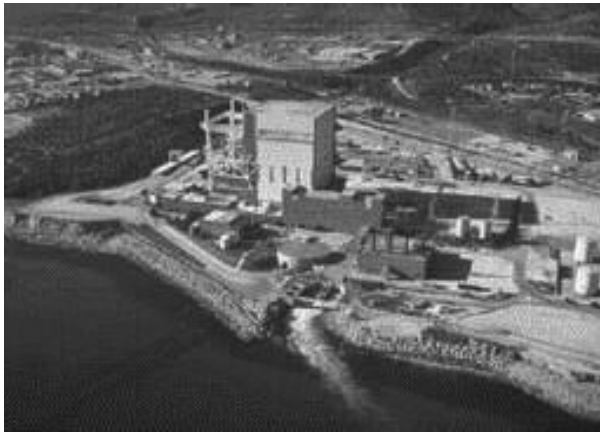
Fig. 2. Decommissioning Vandellós I nuclear power plant in Spain (courtesy of ENRESA).
