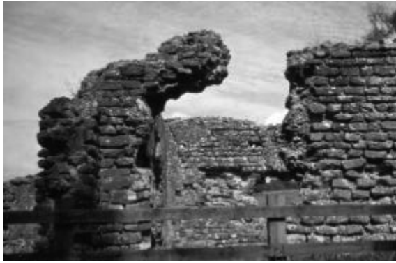
Fig. 8. Typical lime mortar and stone construction from the Roman Fort and Bath House at Glannoventa (Ravenglass, Cumbria, United Kingdom) (courtesy of Nirex).
