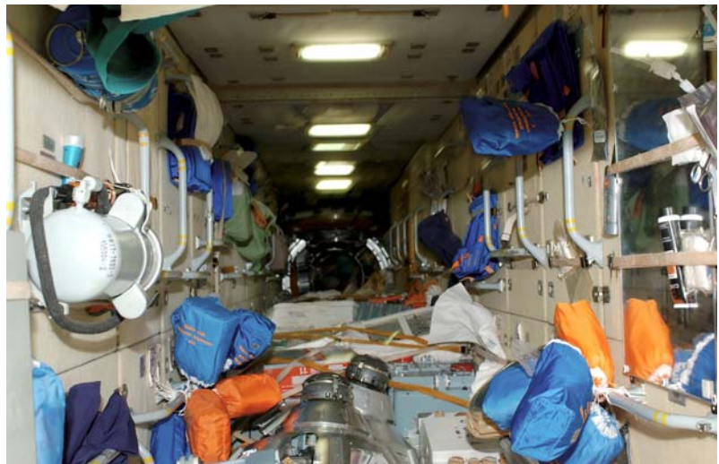
Figure 10-6. ISS010-E-25228 — This view shows supplies and equipment stowed in the functional cargo block (FGB) or Zarya photographed by a crew member on the ISS. (NASA Human Spaceflight Gallery, 2008).
