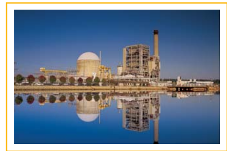
Robinson Nuclear Plant
