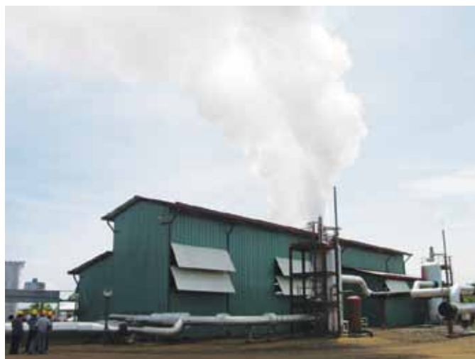
Figure A5.2: San Jacinto Project, Nicaragua: 2 x 5 Megawatt Back Pressure Plant
