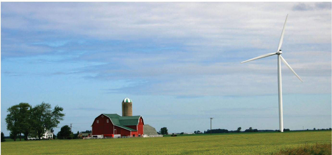
The Harvest Wind Farm near Elkton, MI, is one of several that have been developed to help meet the state's renewable energy requirements. The wind farm represents a $94 million investment and provides enough clean electricity annually to power 15,000 homes (WPC n.d.).
