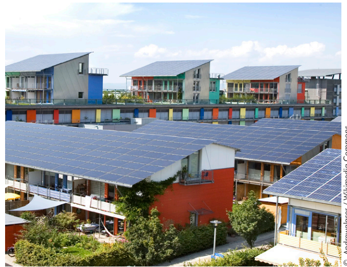
The Solar Settlement in Freiburg, in Germany’s ‘Sun Belt’, is a collection of homes and businesses that produce a positive energy balance and are carbon-neutral.
