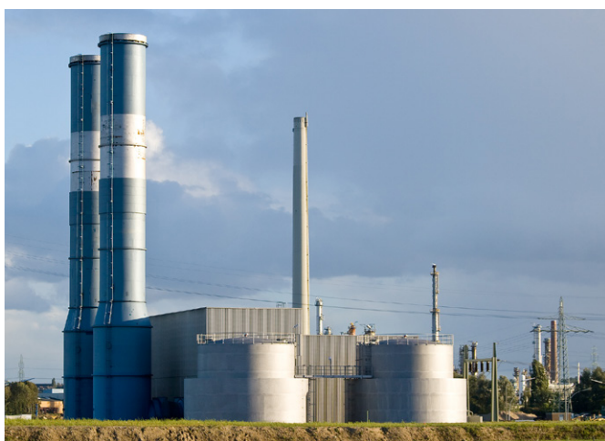
A gas turbine power plant in Hamburg-Moorburg.
