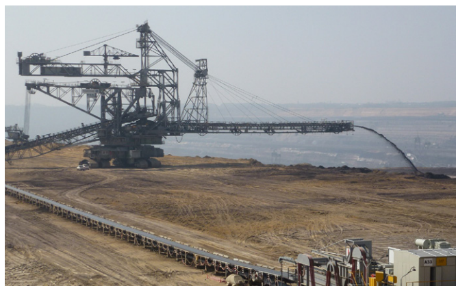
The lignite mine Garzweiler, a 42km 2 surface mine operated by RWE in the state of North-Rhine Westphalia.
