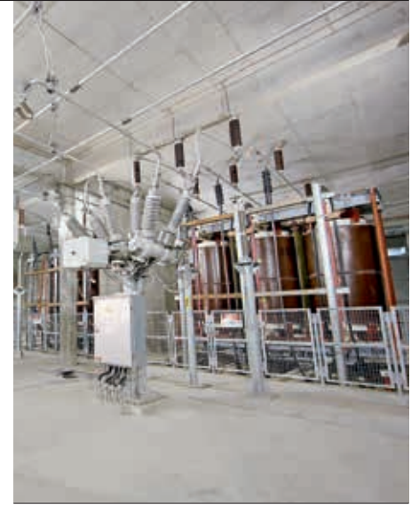
5b PASS M00 72.5 kV SF 6 /air hybrid switchgear
