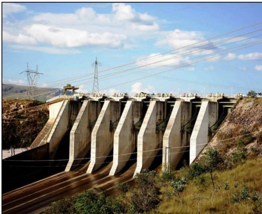
Figure 8: Cheongpyeong Hydro Power Plant 11
