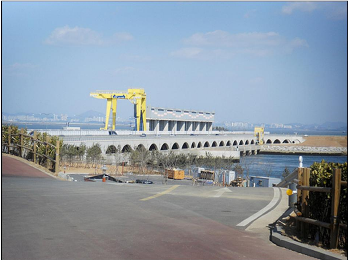
Figure 9: Sihwa Lake Tidal Power Station, construction 13
