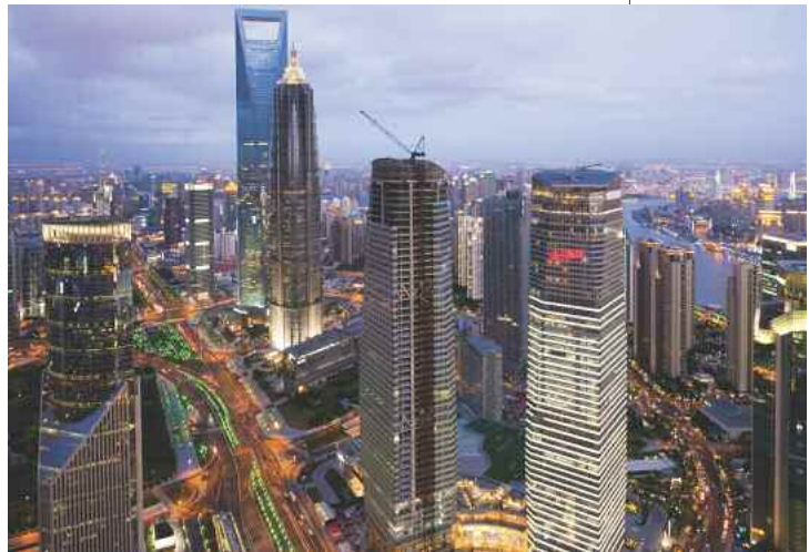
Ongoing construction in Shanghai.
