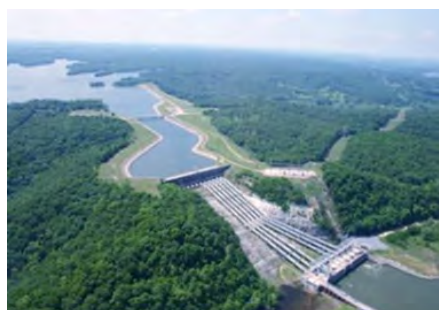
Grand River Dam Authority (GRDA) Salina Pumped-Storage Project, Oklahoma
