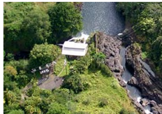
1.1-MW Waiiau Hydro Power Plant on the Wailuku River, Hilo
