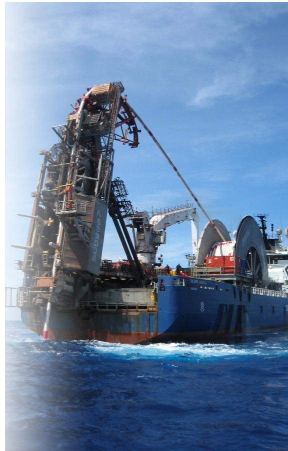
Figure 23: Marine Construction Vessel Installing Flowlines
