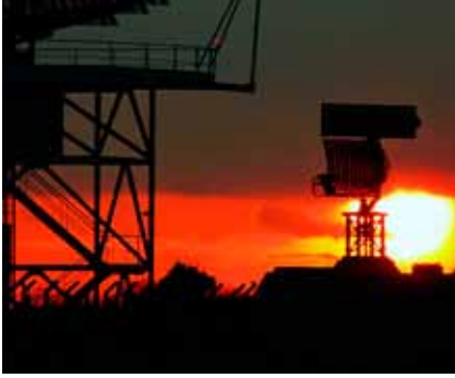
Nav Canada ADS-B tower at Puvirnituq, Quebec on Hudson Bay
