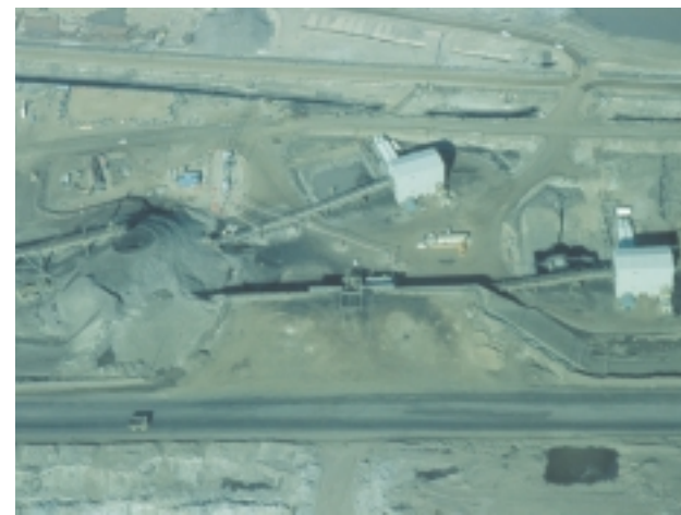
▲ Millennium mine conveyors from air.
