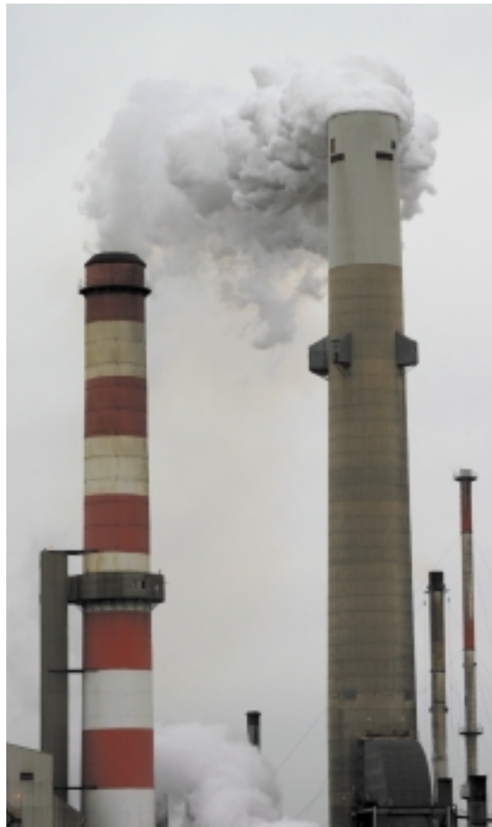
▲ Suncor installed scrubbers in 1996 to reduce SO 2 emissions, achieving a 75% reduction in SO 2 emissions relative to 1990. Regional SO 2 emissions are expected to grow to 295 tonnes per day, which is higher than currently approved emission rates, but lower than the actual emission rates of the early 1990s. PHOTO: SUNCOR ENERGY
