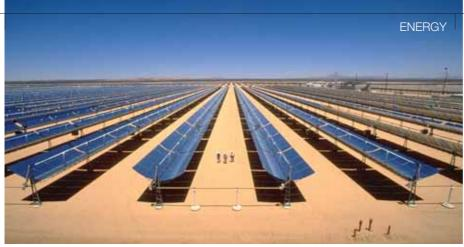
Figure 4 Parabolic trough concentrating solar collector field of the 150 MW (5  $\times$  30 MW) steam cycle solar electricity generating systems at Kramer Junction, California (Source: KJC)
