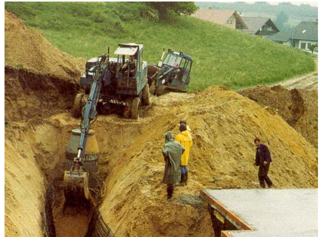
Fig. 7. Ditch collectors - horizontal pipes for extraction heat and cold in Austria.
