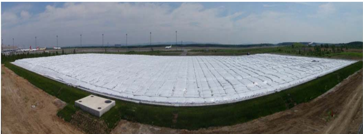
Fig.4 The snow storage at the New Chitose Airport. Here, in May 2010, the snow storage (L: 200m, W: 100m, D: 2 m) is filled up and covered with thermal insulation. (Seppyou, 2012)
