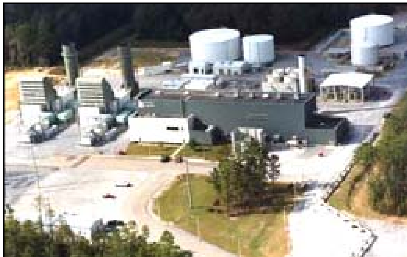
Figure 4-6 Aerial View of an underground CAES plant in McIntosh, Alabama, one of two such facilities operating in the world. The other is in Huntorf, Germany.
