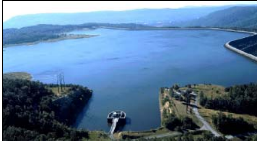
Figure 4-3 Manmade Upper Reservoir of TVA's Raccoon Mountain Pumped Hydro Plant. Operational in 1979, the facility can generate 1620 MW for up to 22 hours.
