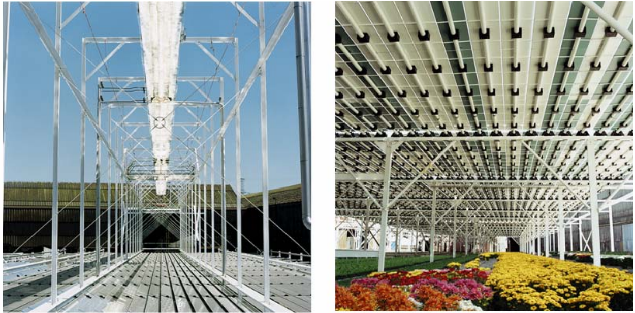
Figure A-45: Energy production above and horticulture underneath a linear Fresnel collector field in a multipurpose concentrating solar thermal power plant. Photos of the collector field by Solarmundo, greenhouse visualisation by DLR.
